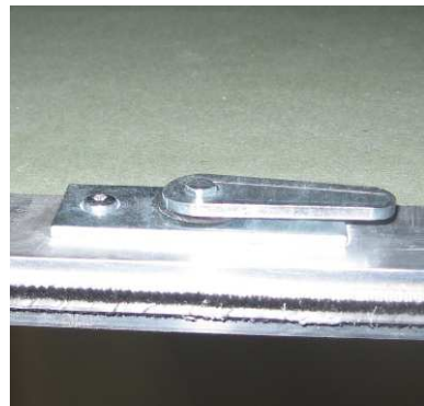
Fig. 8 Aluminium reinforcement for 12.5 mm GKBI panel
