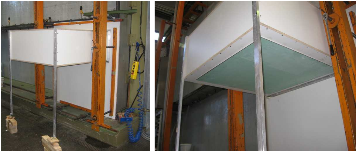
Fig. 12, 13 Test set-up and installation of access panels
